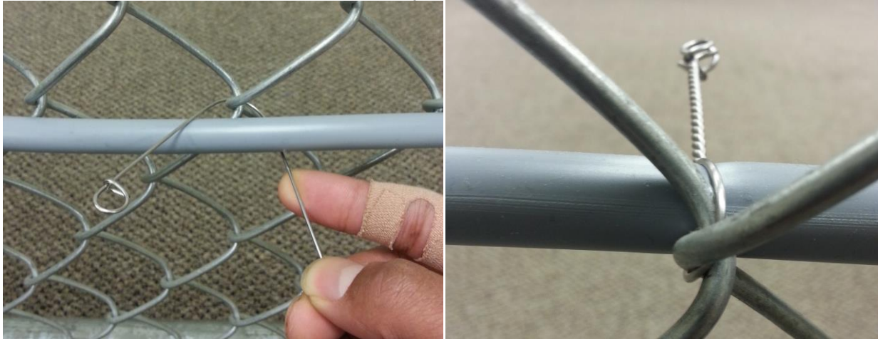
Figure 21a: Observe how the tie fits tightly within the framework of the fence when correctly routed across horizontally adjacent diamonds
