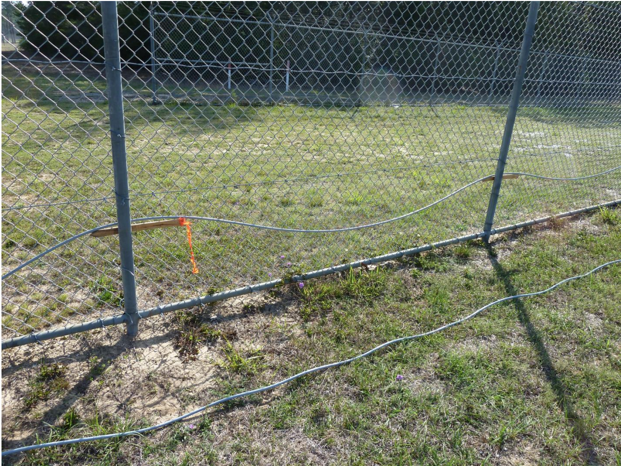
Figure 20: Wooden stakes can be used to create a gap between the fence fabric and the fence post to allow for high security routing of the sensing cable.
