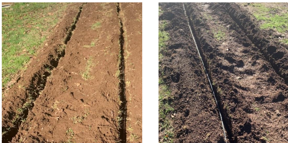
Figure 17. Cable trench examples
