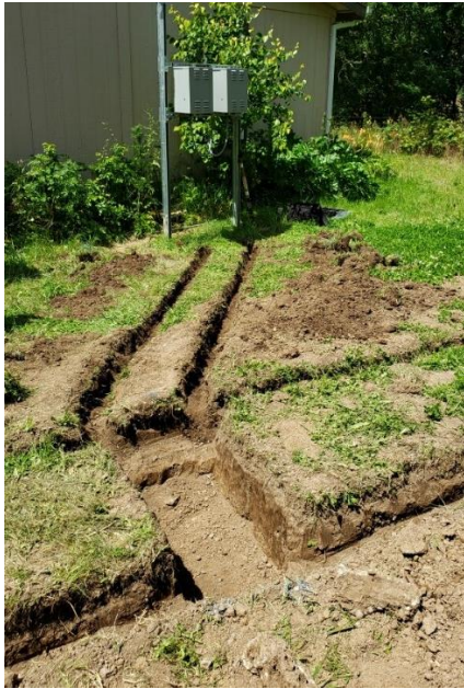
Figure 27. Trenches and Grounding Rod between BSEs
