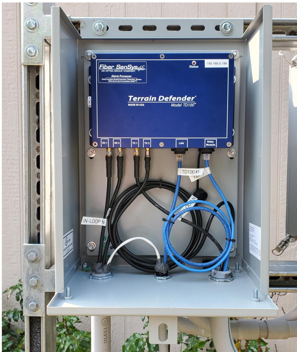
Figure 10. TD100 inside optional TD Outdoor Enclosure
