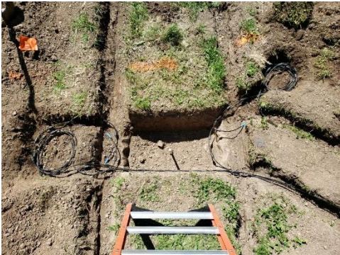
Figure 28. Sensor cables and lead-in cables in place
