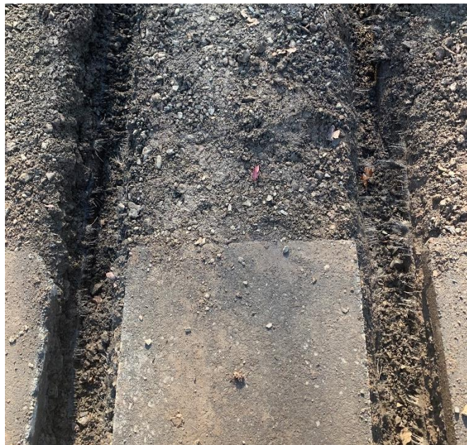
Asphalt to Soil transition maintain 23 cm (9 in) depth
