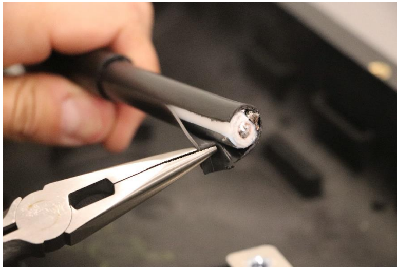
Figure 45. Second jacket slit from cable end to first strip location, outer jacket
