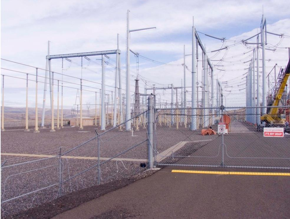
Gates pose a unique problem to fence line fiber-optic sensor cable deployment because they are designed to move. While this does pose a challenge, sensor cable can still be deployed to protect a gate if the following points are kept in mind:
