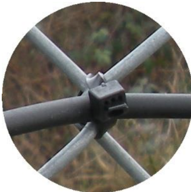
Figure 4-4. Correctly tied through vertically adjacent diamonds.
