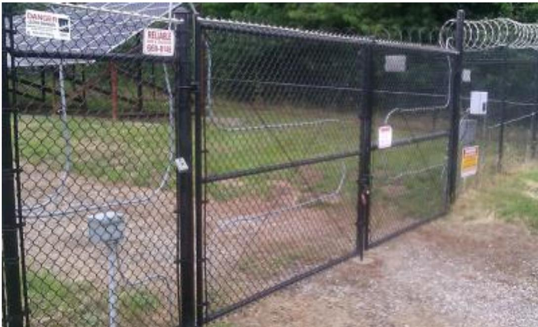
Figure 6: Gate Protection with Fiber-Optic Sensor
